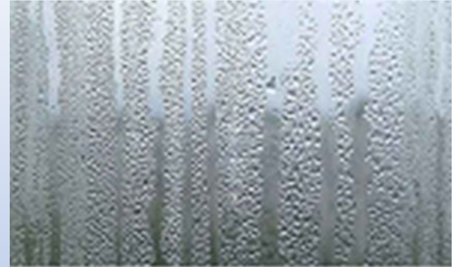
Condensation inside the window
